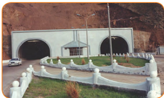
69-rasm. Qamchiq dovonidagi tunnel.
